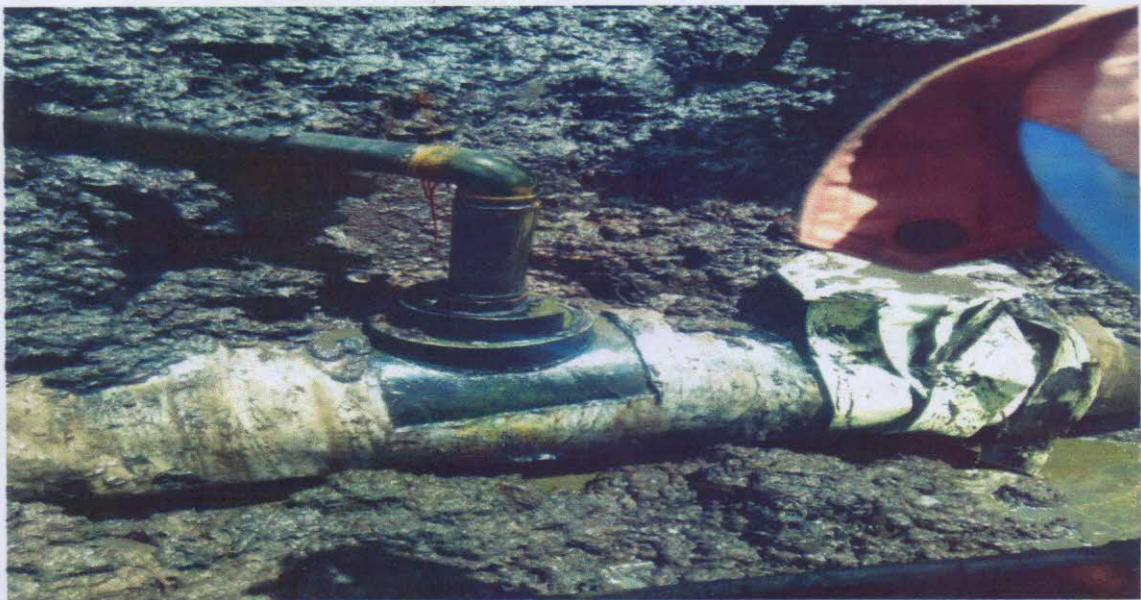
THE SPILL POINT AFTER EXCAVATION
